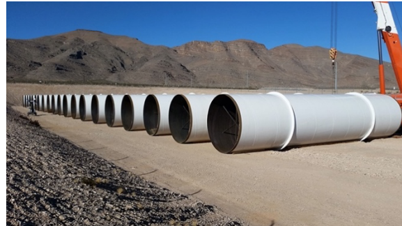
Figure 5: Hyperloop Tube from Steel 6
