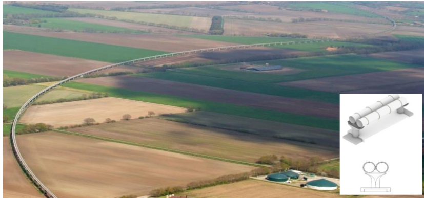
Fig. 1. Part of the northern loop of the TVE's maglev guideway at Lathen, Germany. Continuous loop layout, 32km length. Inset: Elevated Hyperloop bi-tube design [3]
